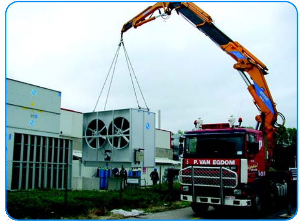
This FXT unit is placed with one lift and ships fully assembled.
